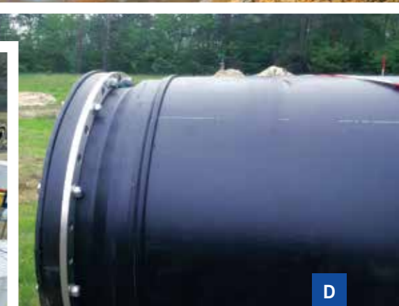
A: The high flexibility AGRU's pipes allow for changes of direction without fittings. B: Visser & Smit Hanab drilled two holes approximately 210 m long underneath the Spree with absolute precision using HDD. C: Visser & Smit Hanab threaded the 220 m long AGRULINE pipeline under the river without, setting a new record. D: A special flange connection with an OD of 1,400 mm, was manufactured by FRANK KUNSTSTOFFTECHNIK GmbH.
