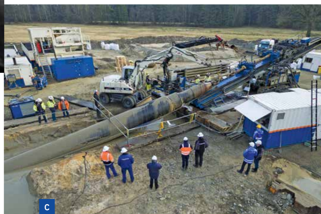
A: The high flexibility AGRU's pipes allow for changes of direction without fittings. B: Visser & Smit Hanab drilled two holes approximately 210 m long underneath the Spree with absolute precision using HDD. C: Visser & Smit Hanab threaded the 220 m long AGRULINE pipeline under the river without, setting a new record. D: A special flange connection with an OD of 1,400 mm, was manufactured by FRANK KUNSTSTOFFTECHNIK GmbH.
