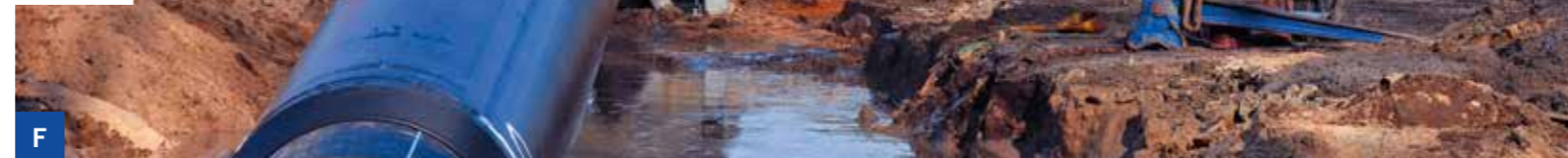
E: The reamer cleared the way for the PE100-RC pipeline. F: The AGRU pipeline adapted itself precisely to fit the exit angle of the borehole as it was pulled in.
